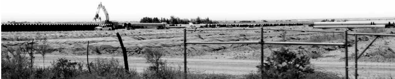
Trans Pecos Pipeline Staging Area | Fort Stockton Tx
