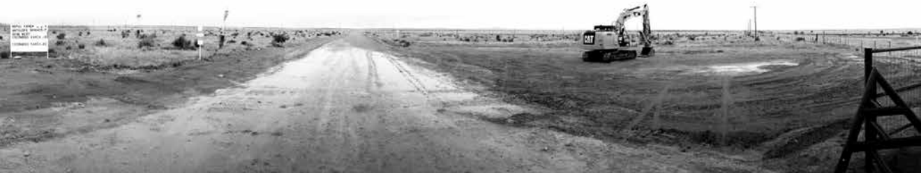
Trans Pecos Pipeline Staging Area Construction | Marfa Tx
